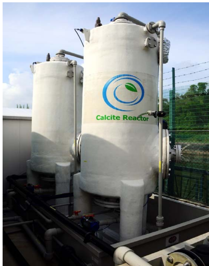
Figure 11 RWM System Calcite Contactors
